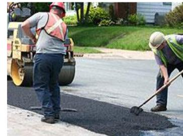
**COVERAGE:** Depth and width of pothole, crack, utility cut etc. will greatly influence the coverage rate achieved. As a rule however, forty pounds of Seaboard BOND-X GREEN High Performance Cold Patch will fill a two inch deep hole, four square feet in size.
